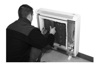
10. Place the heating elements back into their original position. Place the other two rows of storage bricks with the flat side facing out and always on the heating elements supporting tabs.
