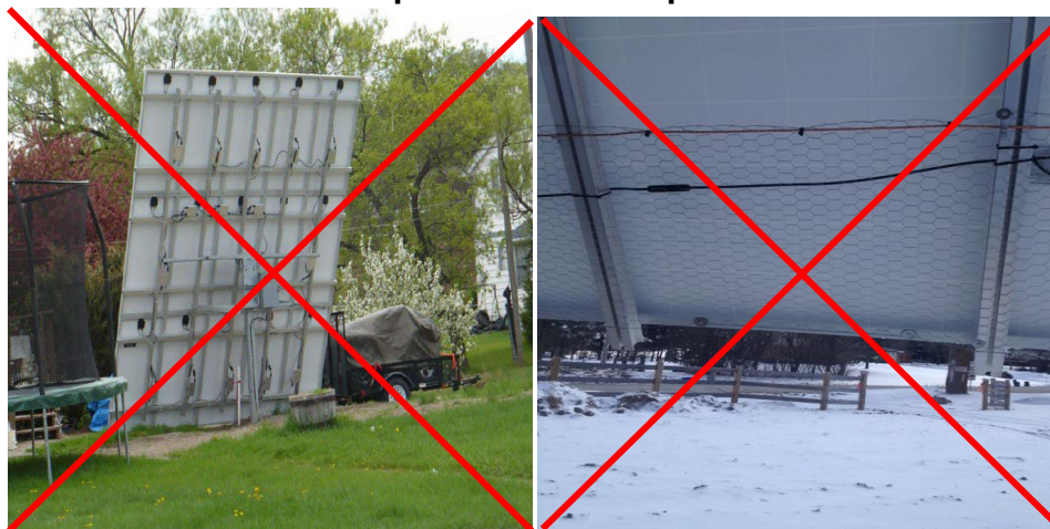
Photo B5 – examples of non-compliant installation
