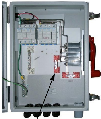
Step 4: Reinstall Positive block
